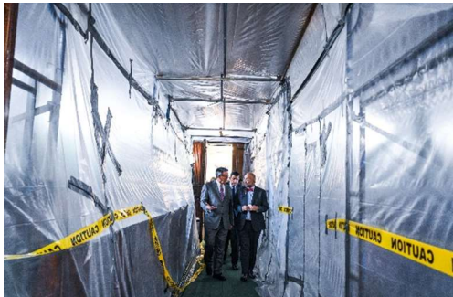
Working Group Co-Chair Hon. Rolando Acosta (left) and member Hon. Shahabuddeen Ally, Administrative Judge of the New York City Civil Court, tour a part of the building under renovation
